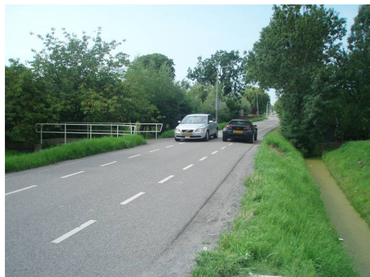
Figures 2-4: Example of Dutch style advisory cycle lanes with single vehicular lane
